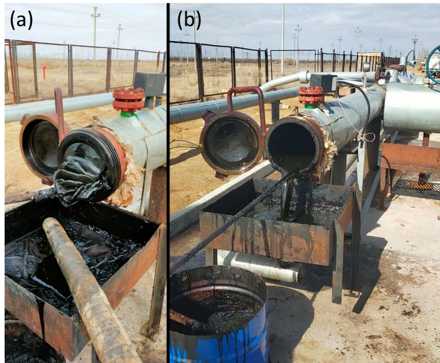
Figure 42 – Example of wax formation on a production line without PPD (a) and free-flowing oil treated with PPD (b)
